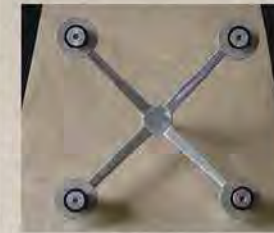
The ground floor vitrine is surrounded with point-fixed glass.
